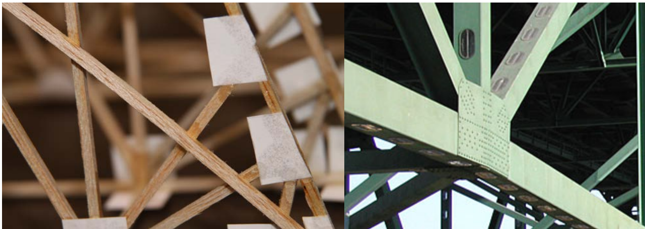
Figure 3a: Gusset plates on a model and actual bridge
